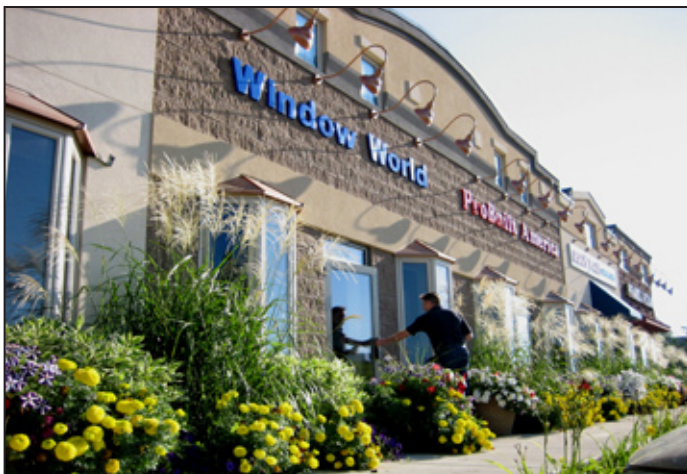
Window World showroom, offices and warehouse
