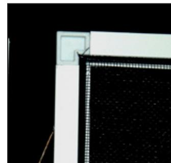
This screen design using rolled form aluminum with keyed corners is flimsy and has unsightly splines.
