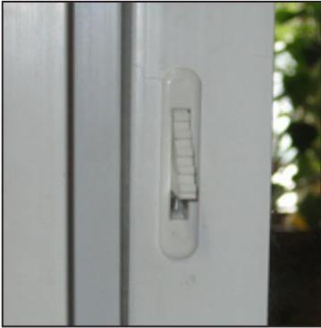
Vent latches are convenient because they can keep the window from opening completely. Police have found the most common way burglars enter your home is through an open window. Keep your vent latches out all the time.
