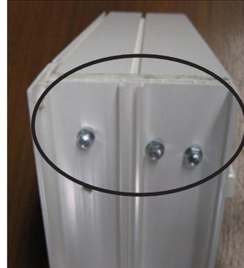
Mechanically fastened corners that are not welded can be weak and not as energy efficient.
